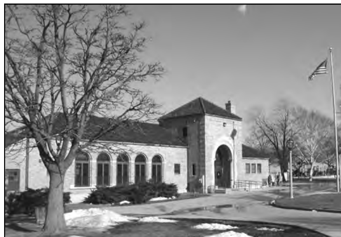
South Shore Park Pavilion home of the South Shore Half Marathon
